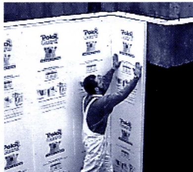
Adhere insulation to clean surfaces, edges tightly butted.
