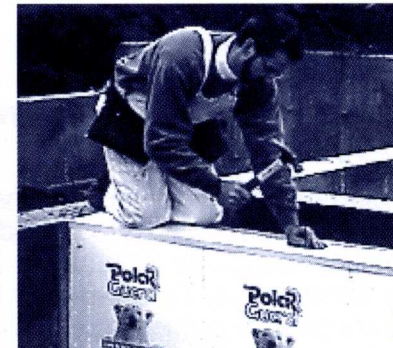
Metal flashing should be installed over foam where it reaches the sill plate.
