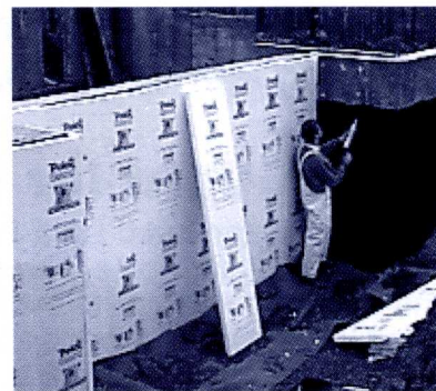
Secure insulation with small spots of panel & foam adhesive.
